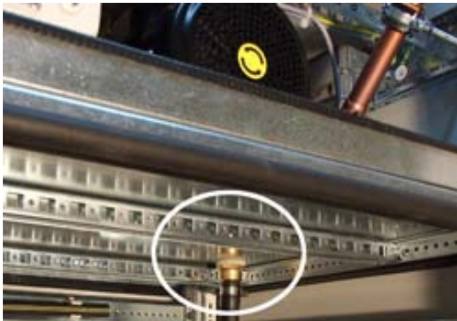
Fig. 4: Drain-tube of water tray
